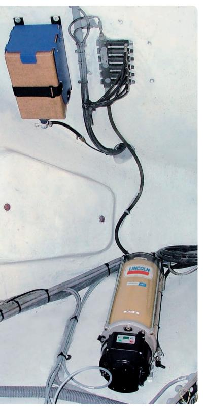
In single-line lubrication systems, a pump feeds the lubricant via the main line to the lubricant metering devices, where it is metered and fed to the lubrication points. The individual lubricant requirements for each lubrication point can be adjusted.
