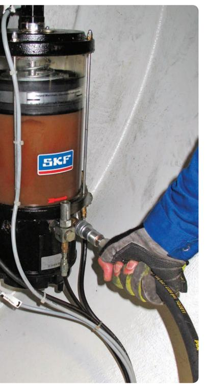
Turbines require large volumes of grease to be dispensed during each lubrication maintenance session. Even though SKF WindLub centralized lubrication systems require minimal maintenance, lubricant must be refilled from time to time. Tower heights and tight working spaces create unique challenges for maintenance workers.
